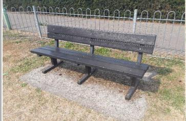
**Finding:** The paintwork on this item has been damaged or worn exposing the metal underneath which is rusting
