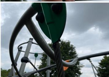
Finding: The ropes/nets are worn/damaged in places
