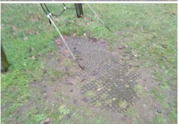
Finding: The grass mats are silted up and the soil is compacted; this may have an effect on the impact absorbing ensure the correct surface qualities are maintained for the properties of the surface
