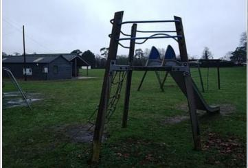
**Finding:** There is/are finger entrapment/s adjacent to the slide entry and the item fails to meet the requirements of BS EN 1176 Part 1 4.2.7.6 Entrapment of fingers
