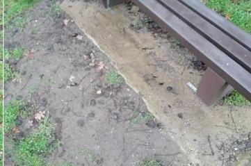
Finding: The surface has eroded and there are trip hazards Action: Reinstate surrounding surface levels to remove the at the edges of the surface
